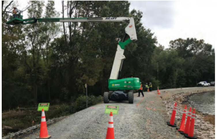
Duke Energy HF Lee Danger Tree Removal
