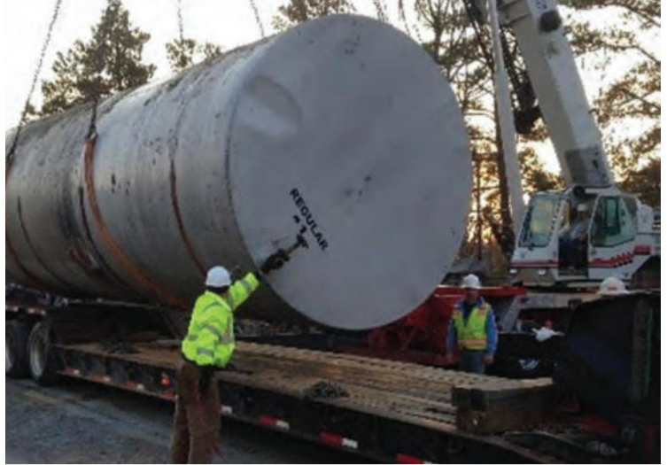
Zava Service Station Demo
